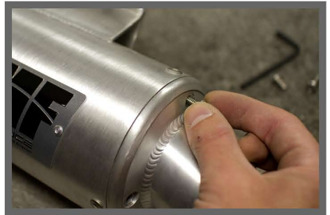
Step 17: Finally, tighten the allen screws on the end cap.
